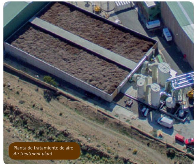
vacuumed air is provided from the inside of the MSW buildings (pit and mechanical treatment buildings) and, if required, through the activation of wall fans distributed on the facade.
